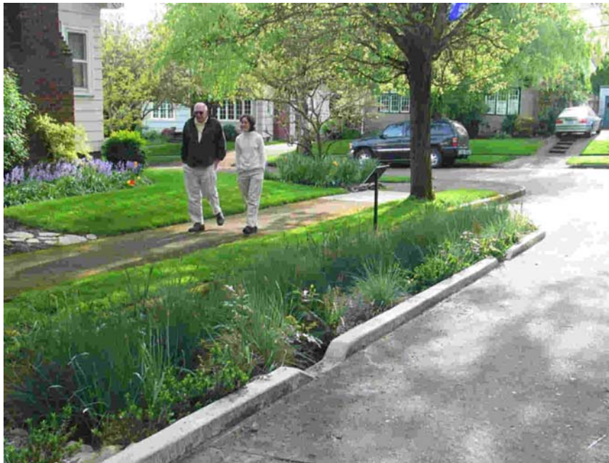
Figure 4.3.2 Stormwater Curb Extension on Siskiyou Street, Portland (Portland Bureau of Environmental Services, 2004)
