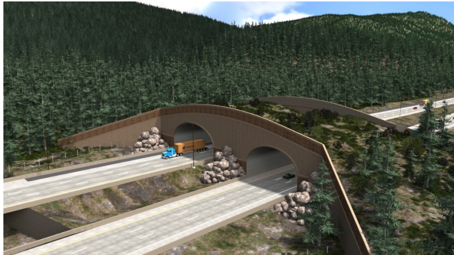
Figure 2-6: Wildlife Bridge over I-90, east of Snoqualmie Pass (Google)
