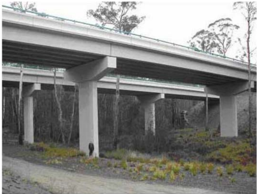
Figure 2-2: The Salty Creek Wildlife Underpass (Abson & Laurence 2003)
