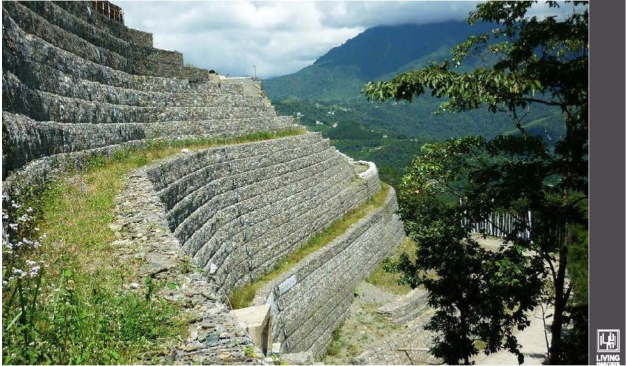
Terramesh Gabion Wall (Rock Face)
