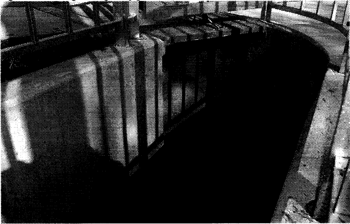
Figure B-7: Leakage through drop gate of Effluent Pond.
