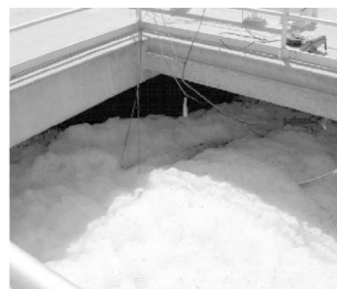
FIGURE 9 Baffle Installation and Its Implications on Foaming and Foam Selection
