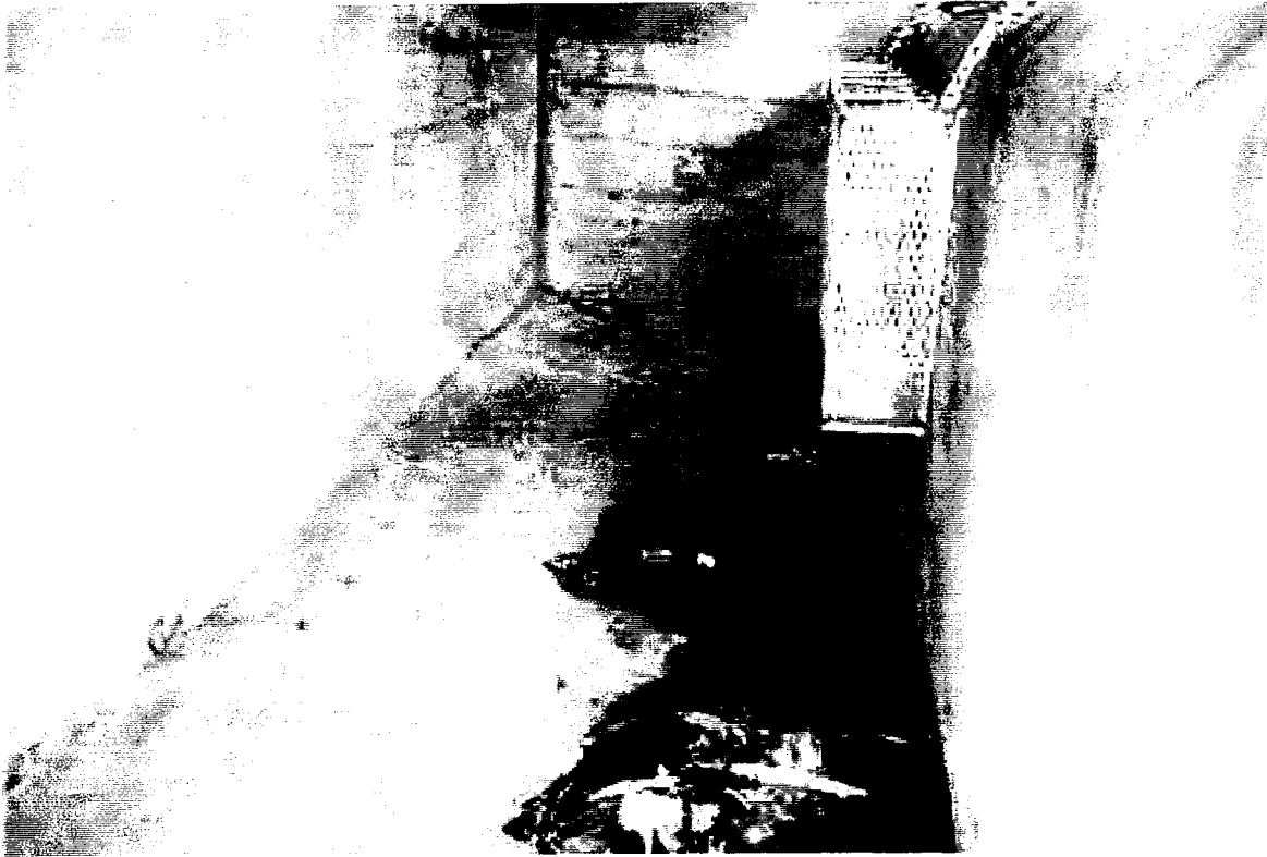
FIGURE 4-15. VIEW INSIDE OF CATCHBASIN SHOWING BASKET INSTALLATION.
