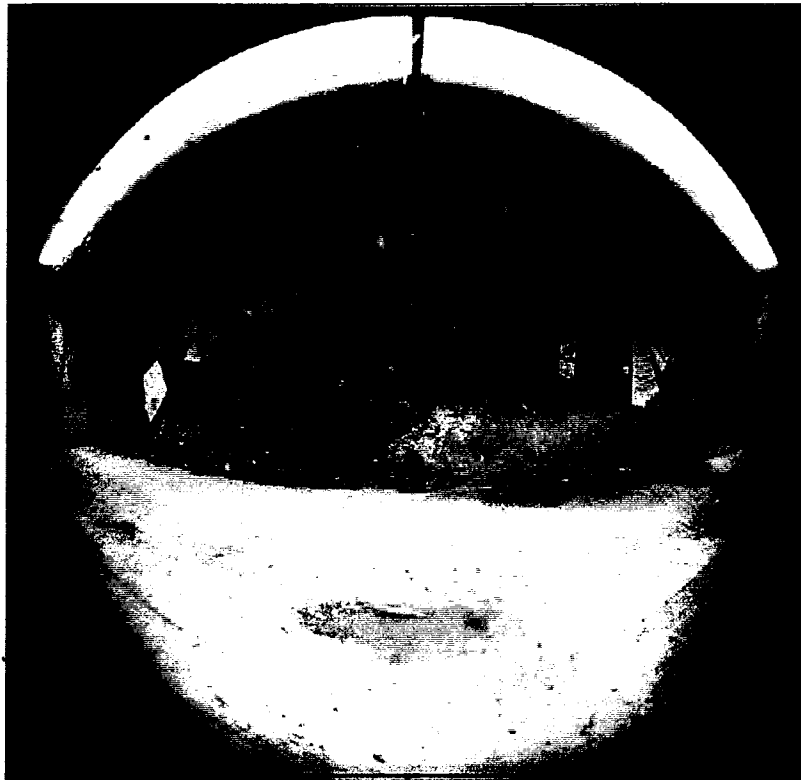
FIGURE 4-8. ACCUMULATED MATERIAL INSIDE CATCHBASIN AT SUNSET PARK AREA, SITE 3 (CONTROL).
