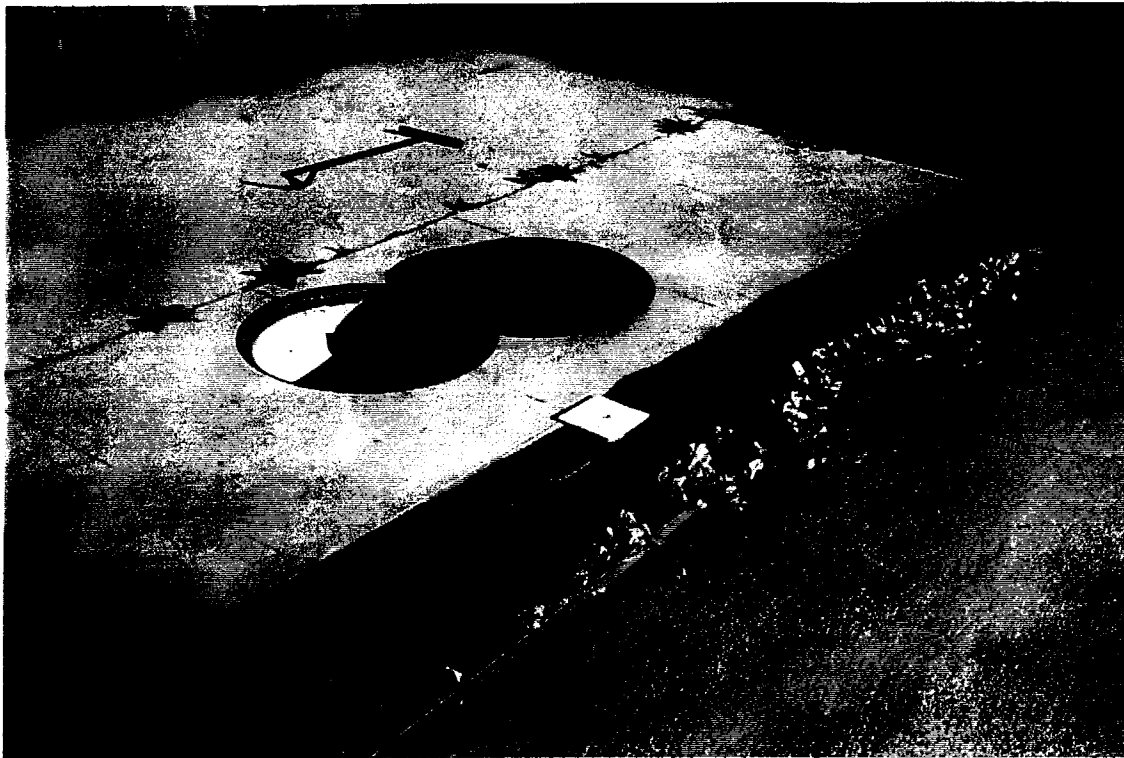
FIGURE 4-9. VIEW OF FRONT OF AB TECH SCREENED CATCHBASIN (SUNSET PARK AREA).
