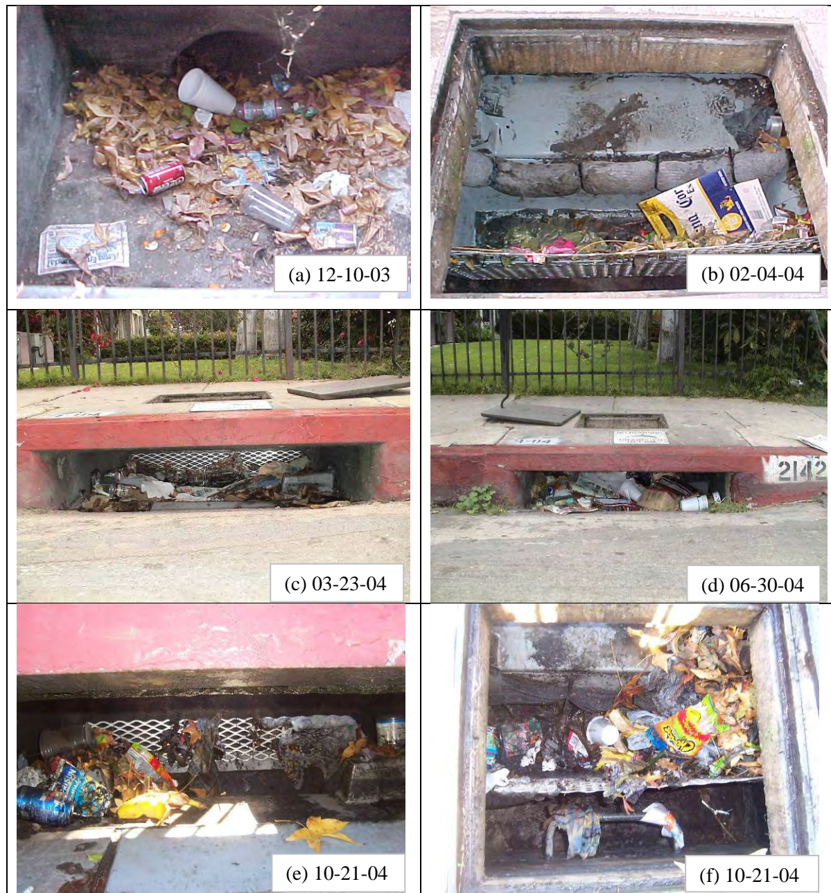
Figure 4-8. Field inspection photos showing the condition of Curb-Inlet Basket at the intersection of 23rd St. and Portland (east side).
