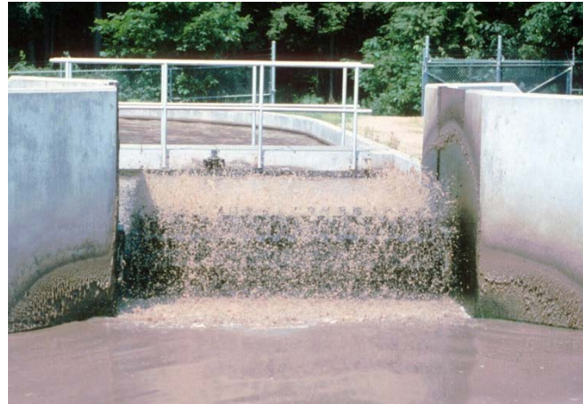
Rotor operating, note the dried spray - a source of odors.
