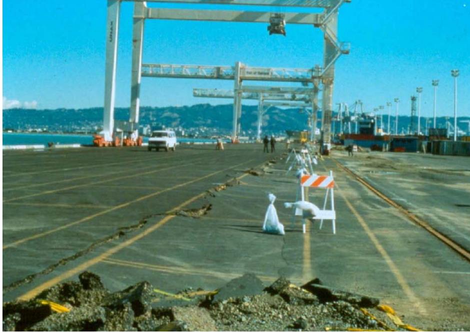
Figure 1.2: Top of the wharf of port of Oakland following the 1989 Loma Prieta Earthquake. The cranes were separated and could not operate as a result of the extension of the wharf (Courtesy of John Egan, Geomatrix)
