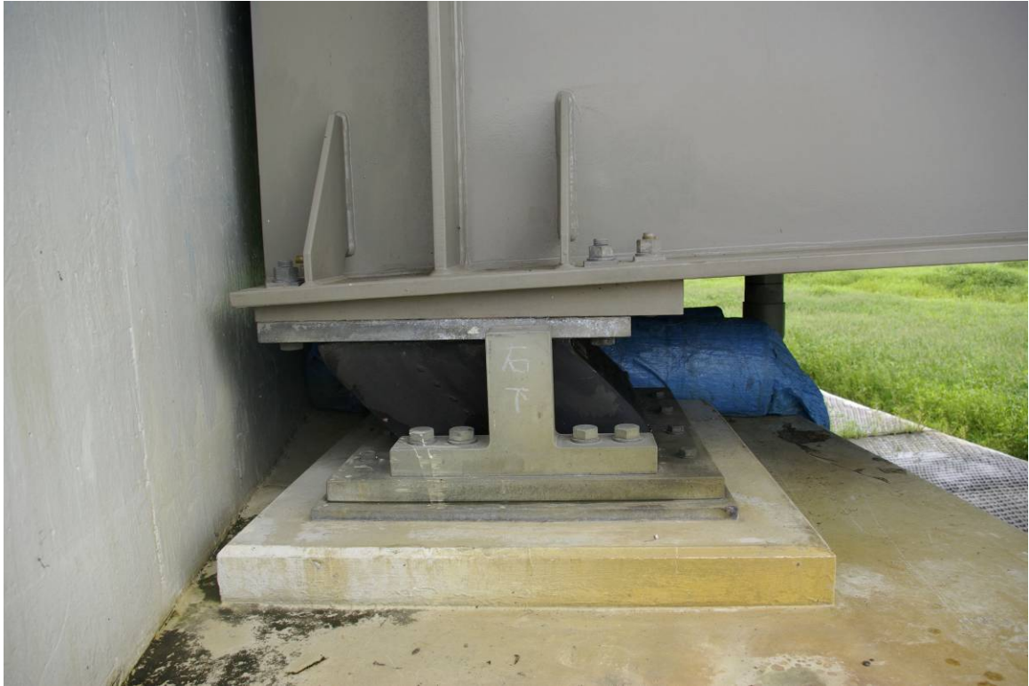
Figure 1.11: Permanent offset in elastomeric bearing at Nagomi Bridge caused by ground deformation during the Niigata Chuetsu-Oki earthquake (Kayen et al. 2007).
