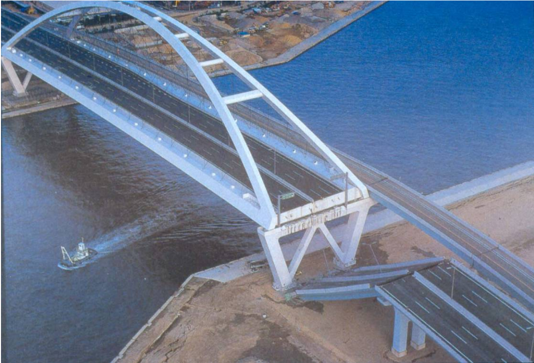
Figure 1.5: Un-seating of the Nishinomiya Bridge as a result of lateral spreading during Kobe, Japan, 1995 earthquake
