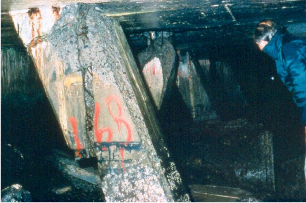
Figure 1.4: Damage to the battered piles supporting the wharf at the Port of Oakland, during the Loma Prieta 1989 earthquake (Courtesy of John Egan)
