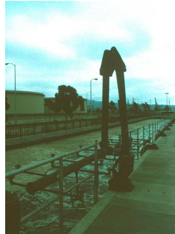
Swing arm in upper Position exposing diffusers
