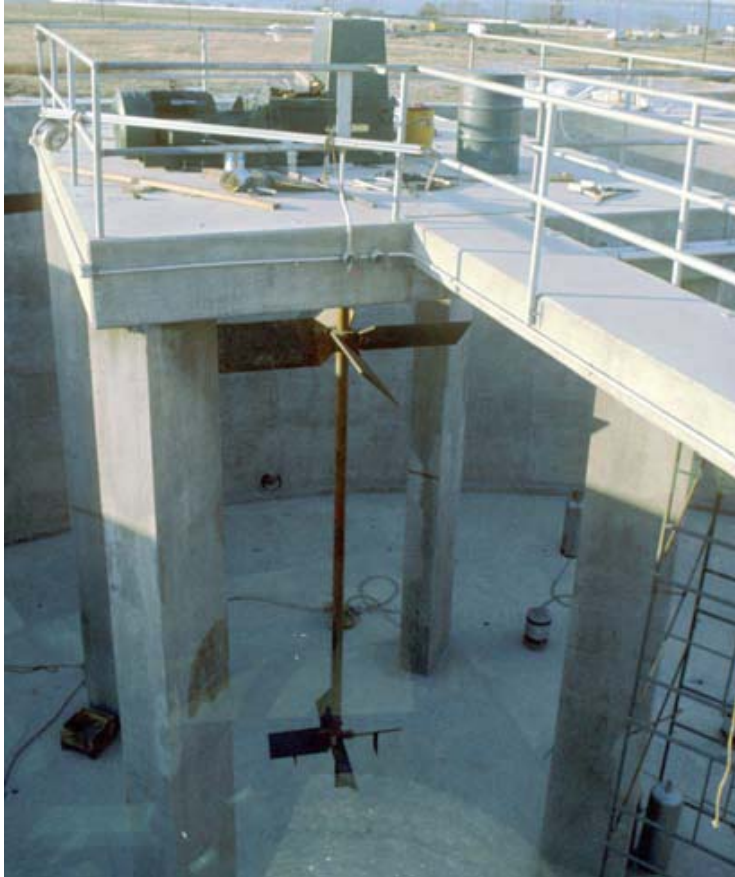
During construction - note that the piers Also serve as anti-vortex baffles
