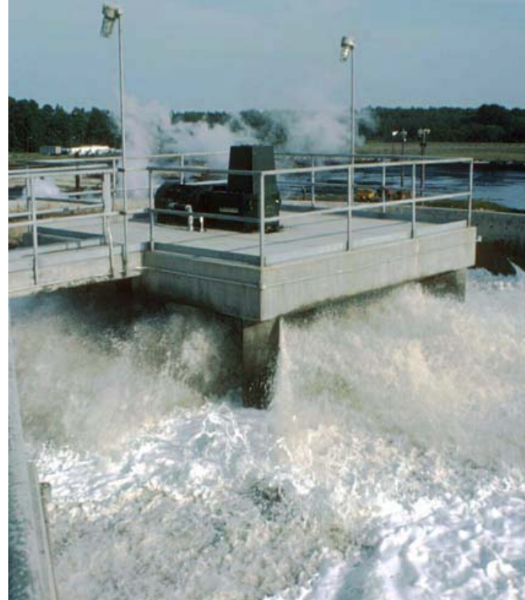
During operation – the spray provides aeration but can causes misting/odor problems
