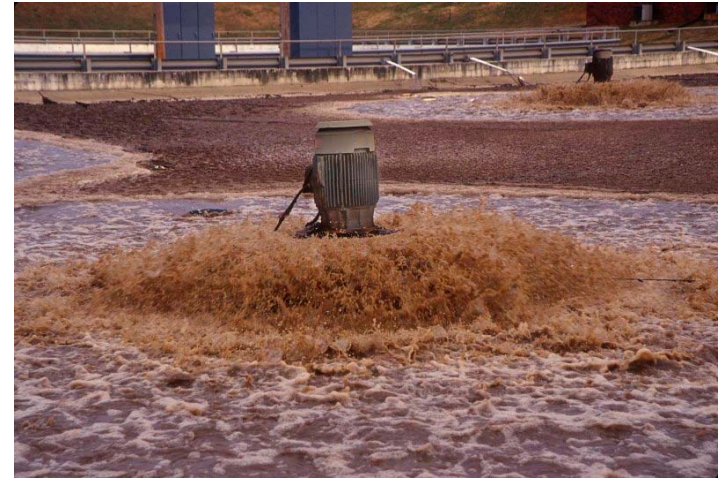
In an activated sludge tank
